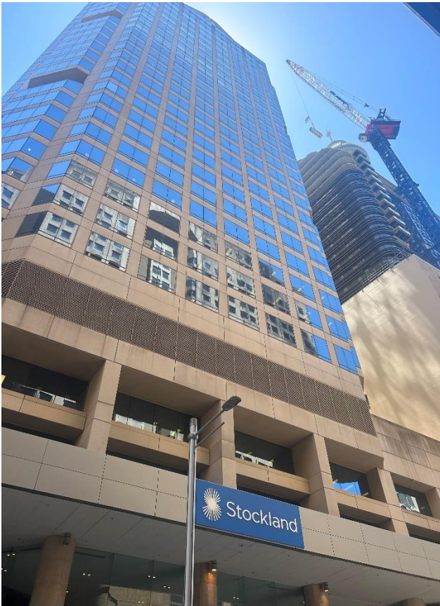
Picture 1 Piccadilly Tower (Castlereagh Street)
