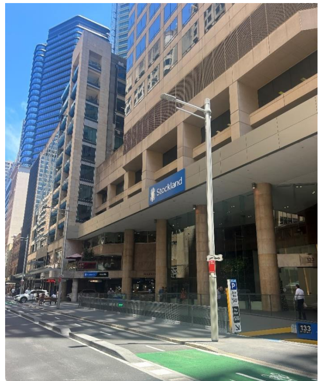
View of vehicular access ramp
